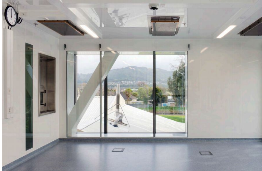
Figure 7: Arcoplast panel system featuring a large, outside-facing window
